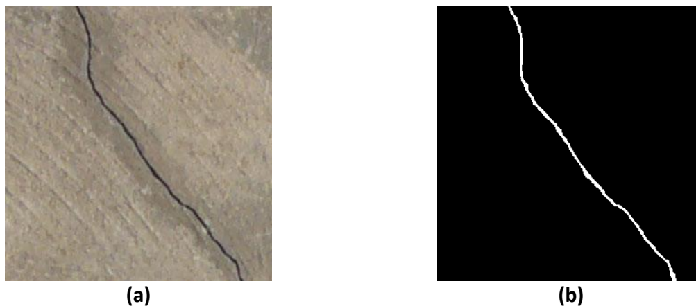
Figure 7. GitHub Crack500 Images: (a) Ground Truth, (b) Cracked Images [82, 83]
